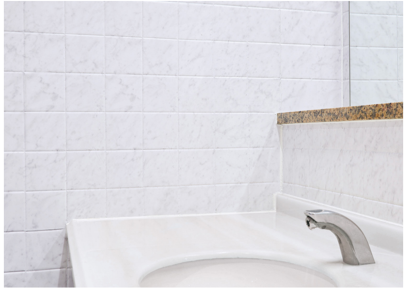
Restroom refurbishment / ST-024TIL
